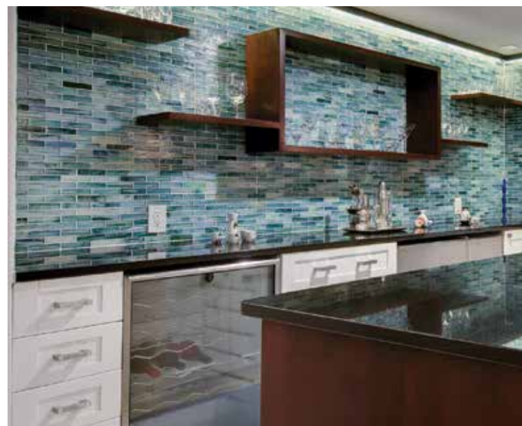
▲ In the bar area of this basement rec room/home theater, wall cabinets and an extremely high bar counter were removed, doors on the existing cabinets were replaced, the exterior of the peninsula was refaced, a new glass bar counter was added and a floor-to-ceiling glass tile backsplash that ties in with the colors in the rest of the room creates a dramatic focal point.
